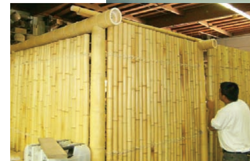
Construction of the new Cedars-Sinai sukkah .
